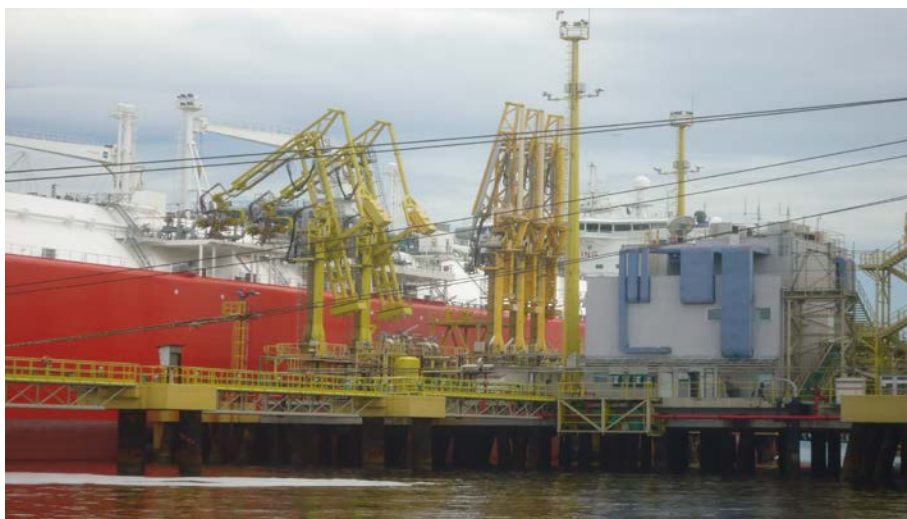
Figura 4. LNG terminal in Guanabara Bay, with detail of the pressurized and air conditioned control block.
