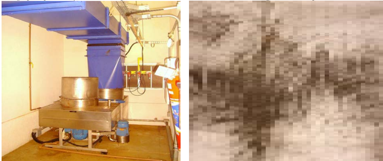
Figura 5. Hydrodynamic precipitator in the capture and desalination of sea air to be blowd into air conditioners, in detail: salt deposited on top of the precipitator and sooty residue of combustion gases from ships.
