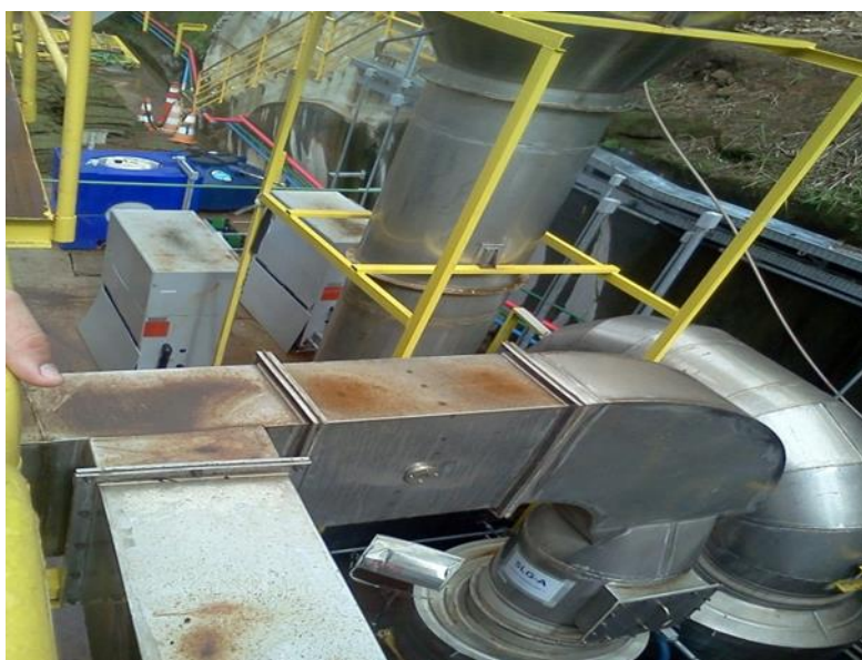
Figure 6. Arrangement with the suction line of gases, hydrodynamic precipitator cooling and condensing the bottom containers of alkaline and waste sludge.
